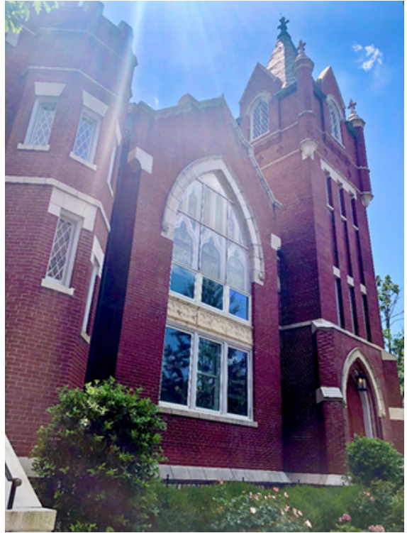
The former Hanover Avenue Christian Church, now The Sydney Condominiums, in July 2020. (Photo by Tre Rockenbach)
