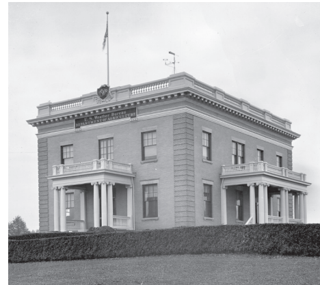
U.S. Weather Bureau Building Exterior, 1918, Cook0569, Cook Collection, the Valentine
