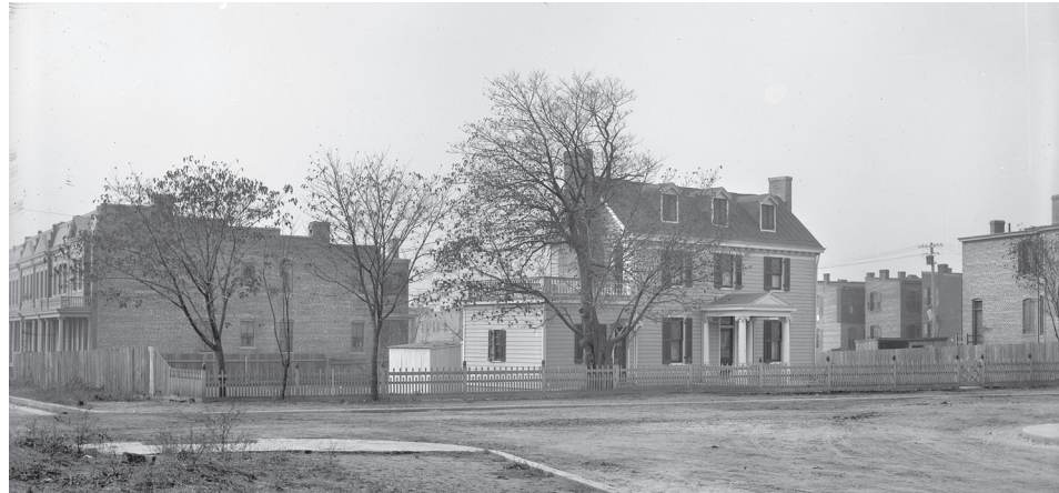
Scuffletown Tavern, Exterior, circa 1905-1913, Cook 0654 Cook Photograph Collection, the Valentine
